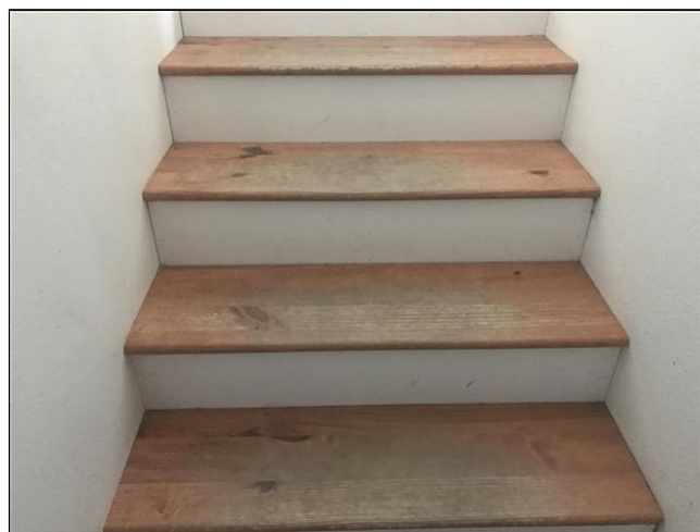
5.2 Item 2(Picture) Damaged hardwood flooring
