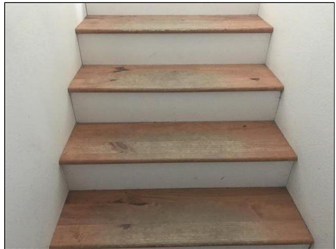
5.2 Item 2(Picture) Damaged hardwood flooring
