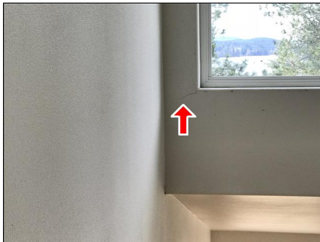
5.1 Item 3(Picture) Settling crack
