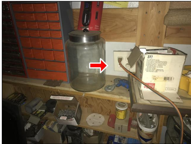
3.6 Item 1(Picture) GFCI outlet needed
