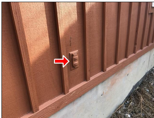
2.7 Item 1(Picture) GFCI outlet needed
