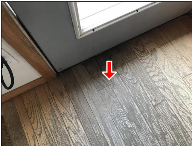
5.2 Item 1(Picture) Damaged hardwood floor
