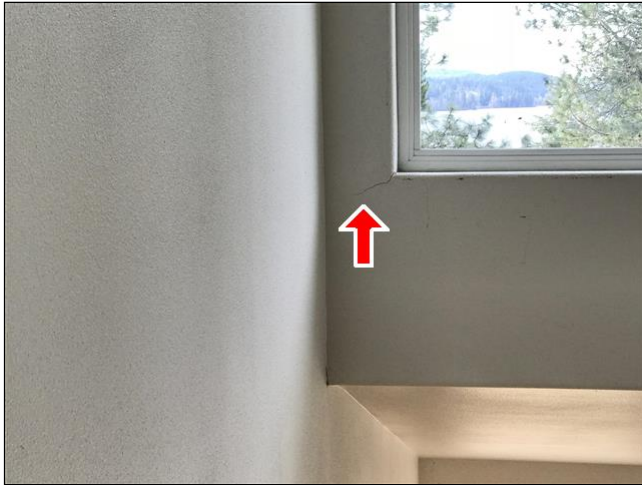
5.1 Item 3(Picture) Settling crack
