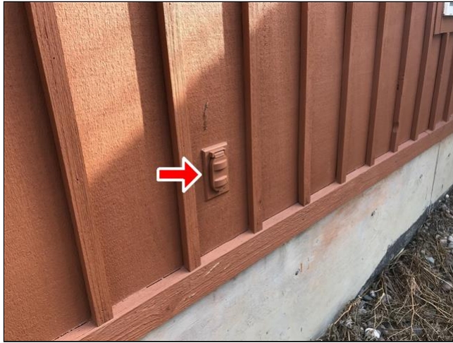
2.7 Item 1(Picture) GFCI outlet needed
