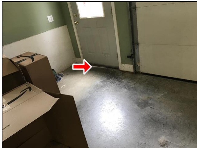
3.3 Item 1(Picture) Visible daylight/missing door sweep
