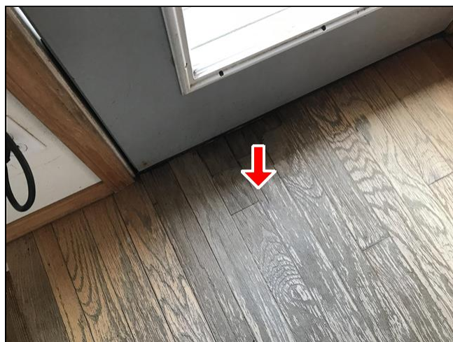
5.2 Item 1(Picture) Damaged hardwood floor
