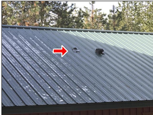
1.2 Item 1(Picture) Damaged/missing vent
