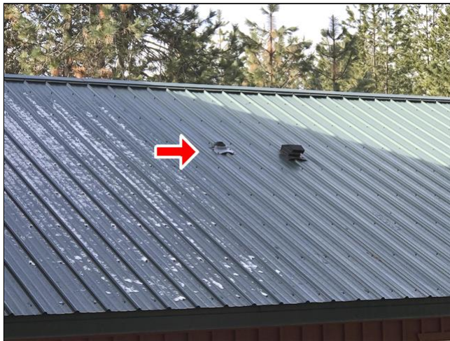
1.2 Item 1(Picture) Damaged/missing vent
