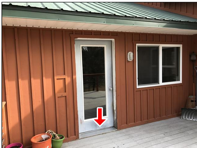
1.4 Item 1(Picture) Splash damage
