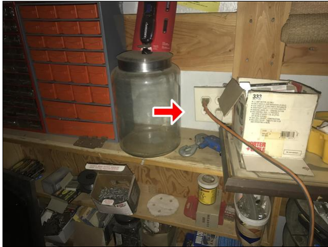
3.6 Item 1(Picture) GFCI outlet needed
