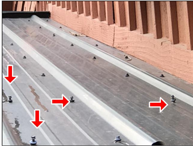
1.0 Item 1(Picture) Loose roof screws
