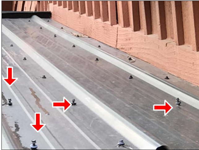
1.0 Item 1(Picture) Loose roof screws
