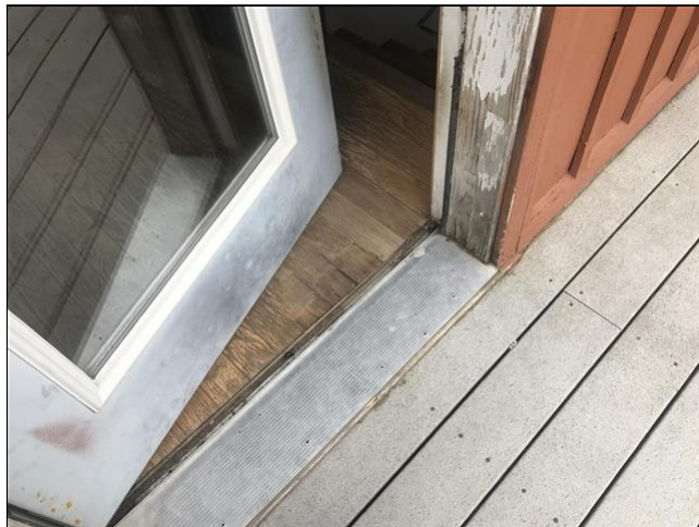
2.1 Item 2(Picture) Splash damage
